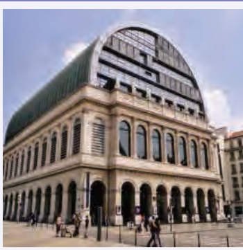
Lyon Opera House / Jean Nouvel, 1993, France
